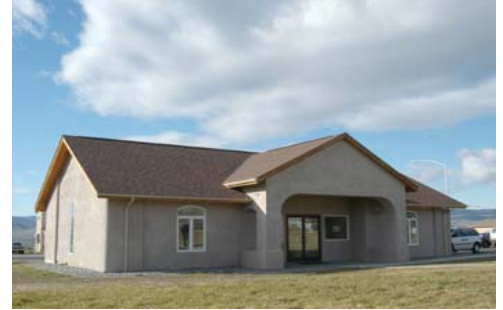
Strawbale walls provide excellent insulation
