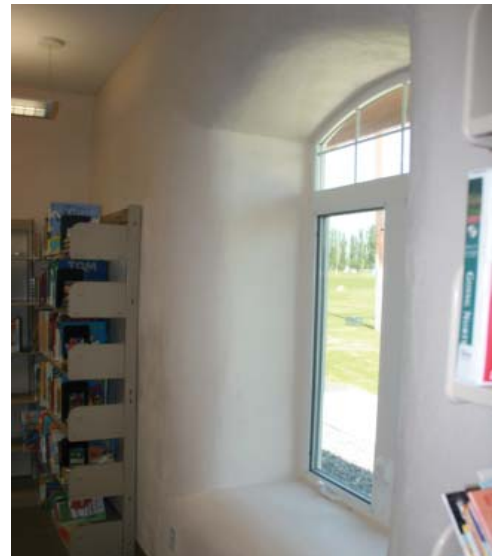
Double glazed, low-e, argon filled windows
