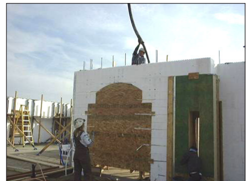
Pouring ICF Walls for greater insulation
